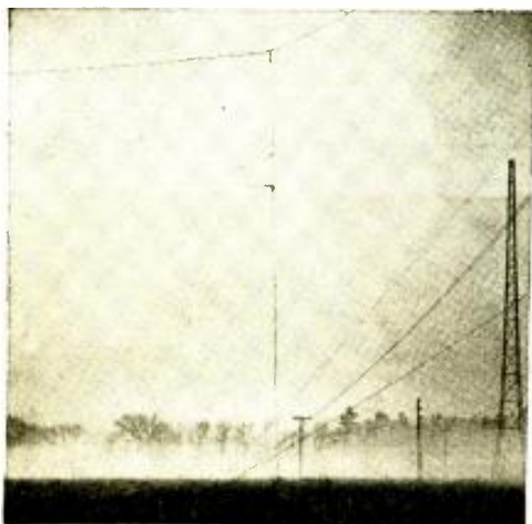
The half-wave vertical doublet aerial at W2XAD, S. Schenectady, today.
