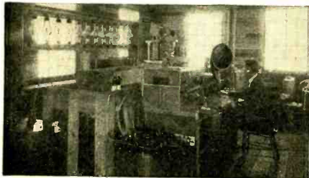
← W2XAF, S. Schenectady, August, 1928. Panels contain crystal control and power amplifier.
