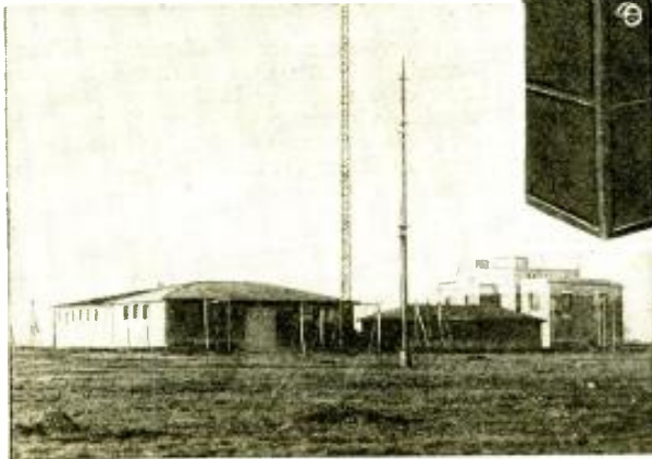
Below—Exterior of the new French transmitting station, showing antenna masts.
